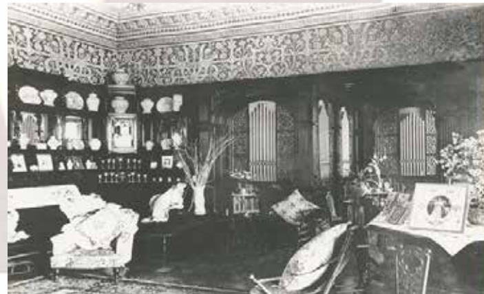
Pipes section of the Aeolian Organ in the Drawing Room c. 1904
